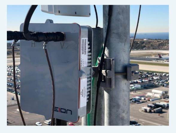
The air navigation service provider for LAX airport has implemented the EION Wireless Radio system as a standard for their wireless infrastructure throughout the airports. This system provides surveillance on the airport surface and during the approach to improve the air traffic controller's ability to manage airport traffic regardless of visibility and weather conditions.
