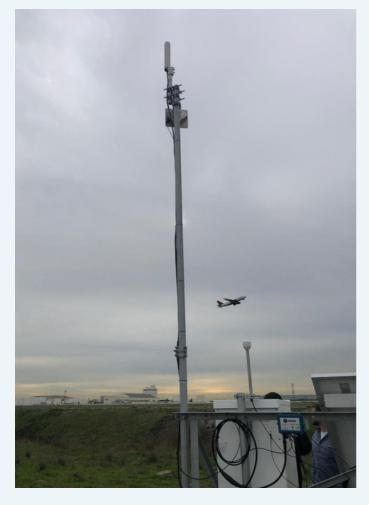
The wireless network at LAX airport consisted of four EION 5300-58 base stations and 51 EION 1130-58 remotes, which cost around 200K USD. The project was implemented by two installation teams and two professional wireless network engineers working in parallel.
